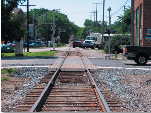
Fig. 55. Ann Arbor Railroad Right-of-Way at Liberty Street
